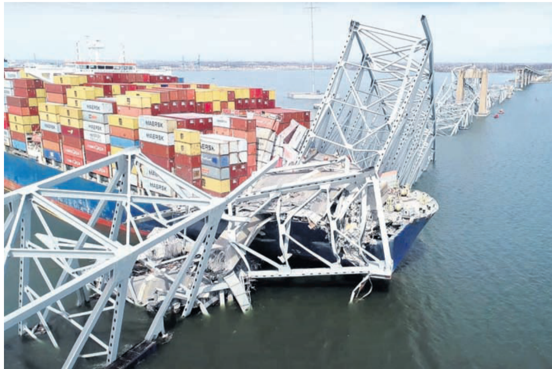
In this image taken from video released by the National Transportation and Safety Board, the cargo ship Dali is stuck under part of the structure of the Francis Scott Key Bridge after the ship hit the bridge, Tuesday, March 26, 2024, in Baltimore.
